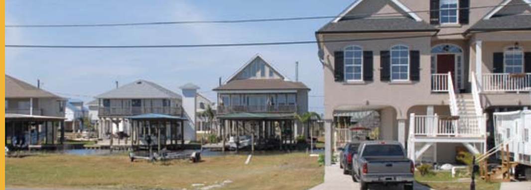
April 4, 2006 — This community in Empire, Louisiana, received no damage from Hurricane Katrina because all homes are built above the floodplain. Marvin Nauman/FEMA
